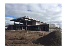
We are past the halfway point of completion for the new Multipurpose Building at Marsh! Construction crews are currently working on making the building weather tight. All interior walls have been framed with metal studs. In the next month, we will observe completion of roofing, stucco and windows and doors.
